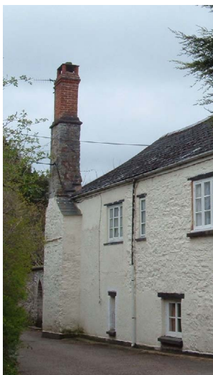
5 Massive external stone stack with brick extension
