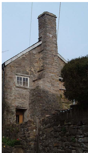
4 Massive external end stack with haunching
